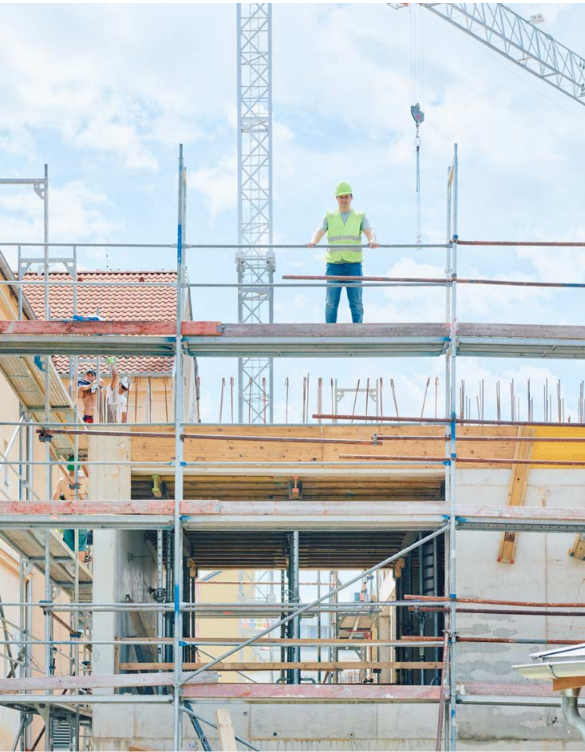
Pohořelice Primary School. A new extension with three above-ground floors and an attic section is being built for the existing primary school building in the town centre. Pupils will receive six new specialised classrooms for studying natural sciences, foreign languages and digital technologies, as well as a new school kitchen with a modern canteen. The photo of the school building under construction shows its project manager, Ing. Michal Kužel.
