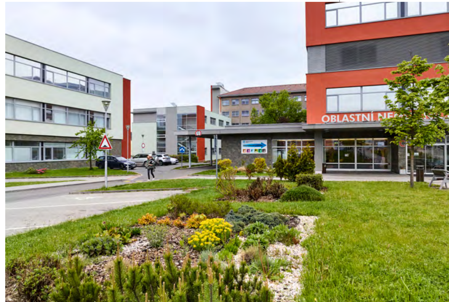
↑ The construction of a new children's ward at Příbram Hospital substantially contributed to improving the quality of care, as well as supported the city's infrastructure. Winning PS secured the general delivery. The picture shows a building in the middle.
