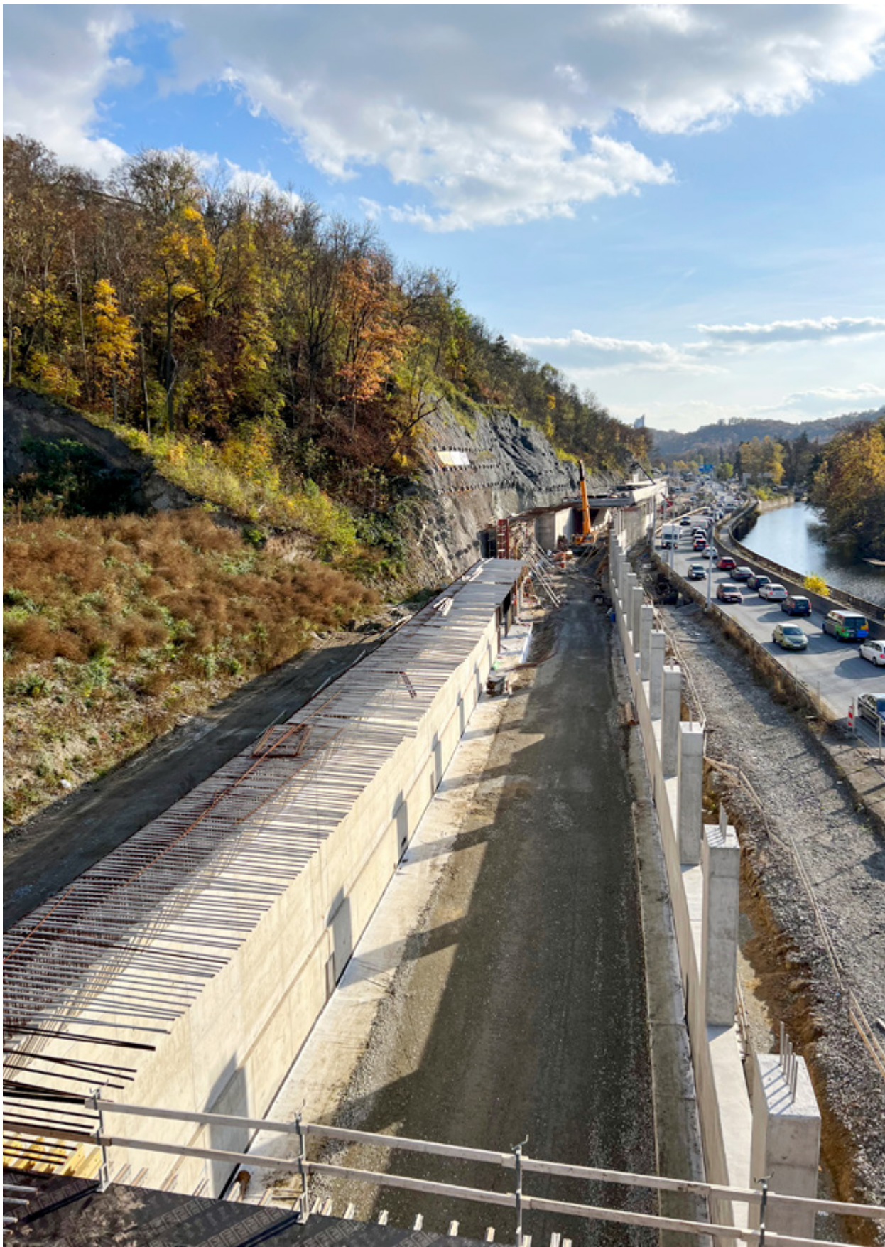
The large Brno ring road has a new 350 m long section leading from Královo Pole towards the exhibition centre. Reinforced concrete structures were supplied for it by Winning PS Pamstav. The two-lane gallery with one column, which is 7 metres in height, consists of 20 expansion units. Construction took a year and a half.
